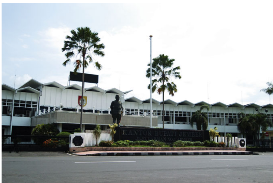
Fig. 29.9 Office of Jember district government
