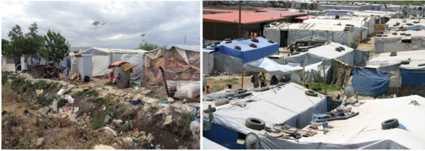
Fig. 5.7 Informal tent settlements of refugees from Syria in the Lebanon. Refugees require space to meet their housing needs. The tent settlements do not meet the required standards for human dwellings and are causing ecological damage. The increasing number of people living in precarious conditions and scattered across the land is determining a loss of landscape character and quality. Photographs Maria G. Trovato
