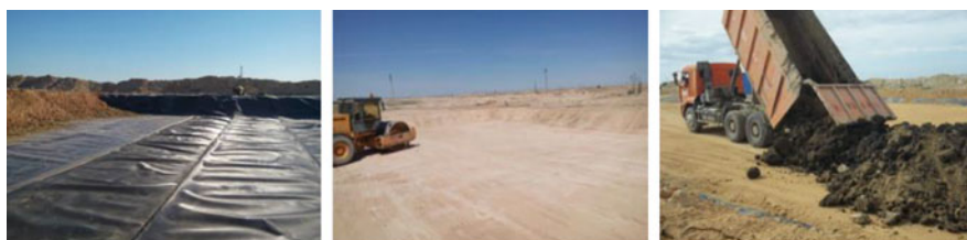
Fig. 26.2 Construction of the bioremediation platform
