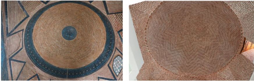
Fig. 1 Patterned brick domes Left : Sahib Ata Hankah, Konya (1283–93) Right : A vaulted room from Karatay Madrasa, Konya (1251–1253)
