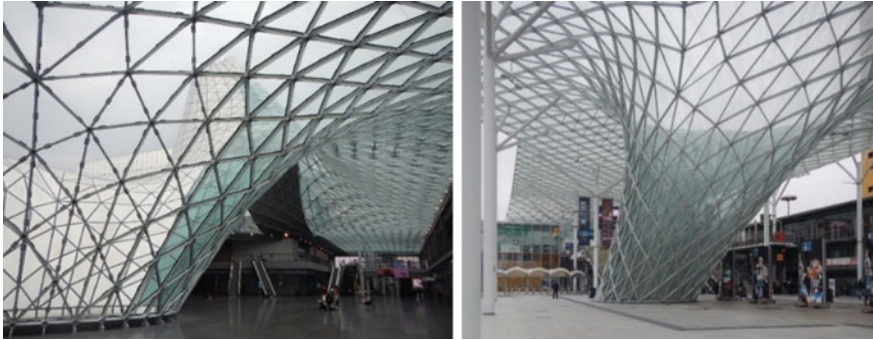
Fig. 8 Drawing survey at the reticular structures in the triangular tessellation roof of the Fieramilano vault gallery (picture of the Author, with courtesy of: Accademia Fondazione Fiera Milano)
