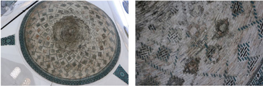
Fig. 7 Patterned brick dome and details from the brickwork from Taş (Aladdin) Mosque in Çay, Afyon (1258)
