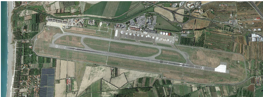
Fig. 5. Lamezia Terme International Airport.
