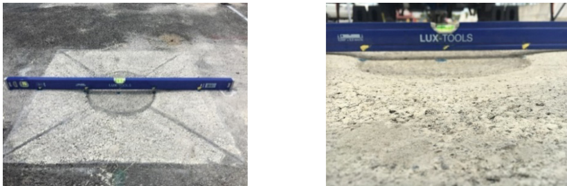
Fig. 3. Rutting at the end of APT tests
