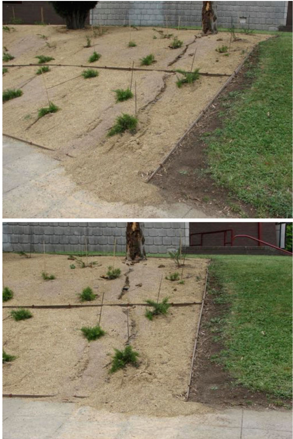
Fig. 12.15 Erosion resulting from concentrated, downslope-directed stemflow. The most prominent stemflow scour, which resulted in the incision of a rill channel, was the result of stemflow from a small Eucalyptus sapling visible at the top of each photograph. Scour downslope of several other plants can also be seen. Both photos show the fan of sediment deposited on a cement path at the base of the steep garden bed. Monash University campus, Melbourne, Australia (Photos: author)
