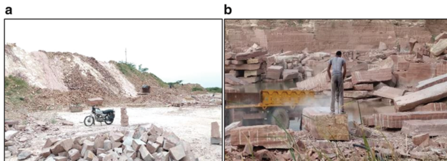
Fig. 5.4 (a) Dumping of waste slurry and scrap stone resulting in artificial mountain of waste (5–10 m in height) (b) Dry drilling in the stone strip using a jackhammer without any safety mask or equipment
