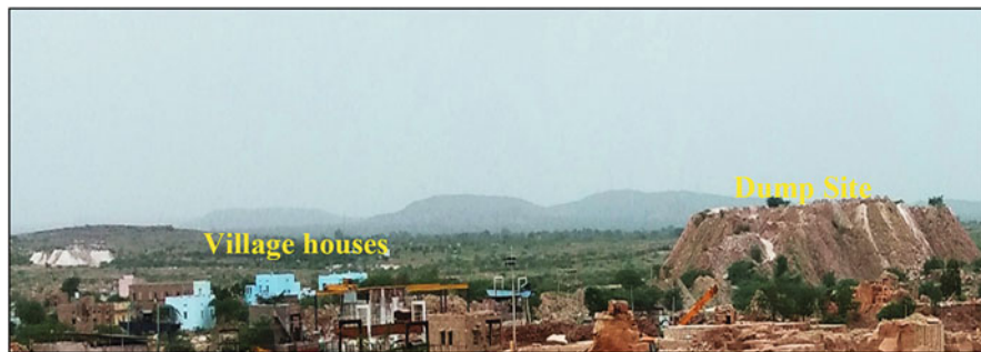
Fig. 5.5 Location of dumpsite close to village houses (150–200 m away, the height of dumpsite is approximately 8–10 m, near village ‘Shiv Sharnon ki Dhai’)
