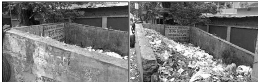
Fig. 8.2 Stationary waste containers used in Kharagpur
