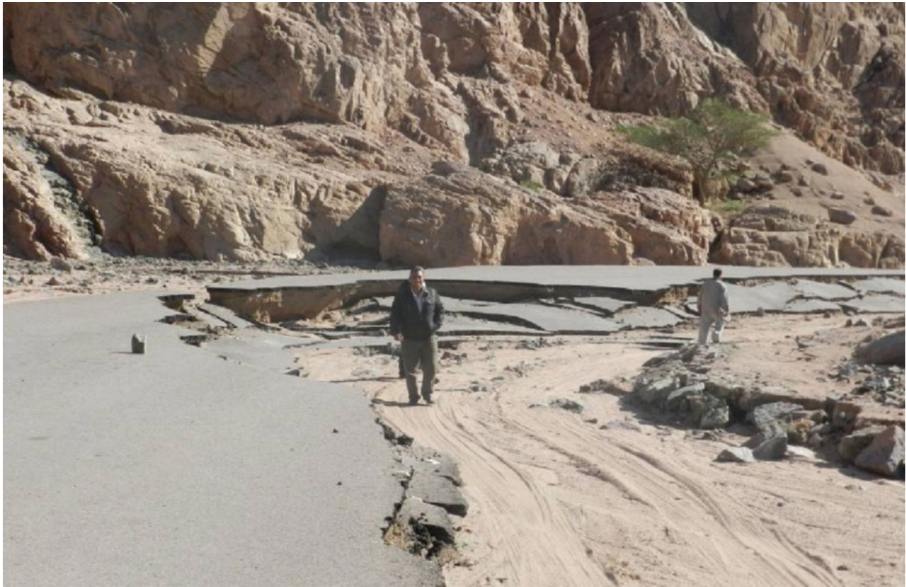
Fig. 4 A photo showing the sabotage affecting the main road to Dahab City, which is caused by the rigorous flash floods of W. Dahab Watershed
