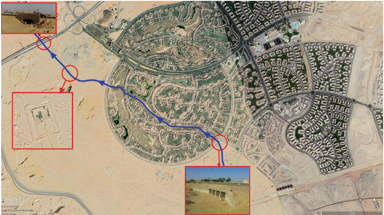
Fig. 15 Madinaty channelized wadi with four vents entrance culverts draining to a smaller culvert under Suez road and temporary detention pond
