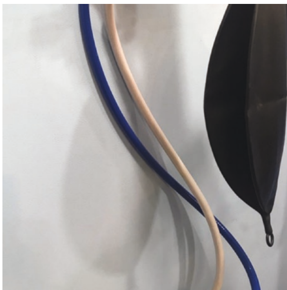
Fig. 4.23 Figure showing color coding of tubes—blue for nitrous oxide and white for oxygen
