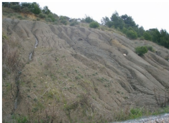
Fig. 12.1 Marl degradation on the cut slope surface at the Adriatic Coastal Road in Croatia. Location: Podstrana, Croatia. (Mišćević and Vlastelica 2012)
