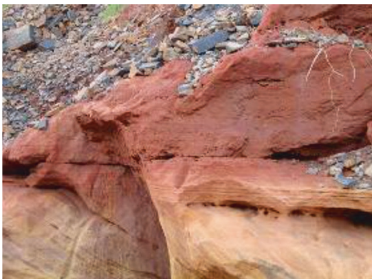
Fig. 5.10 Erosions in sandstones foundation due to seepage (Photo E.L. Pastore)
