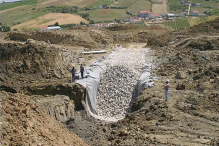
Fig. 4.25 Detail of a drainage trench
