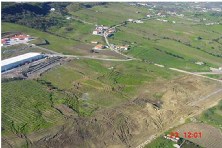
Fig. 4.24 Aerial view of the unstable area
