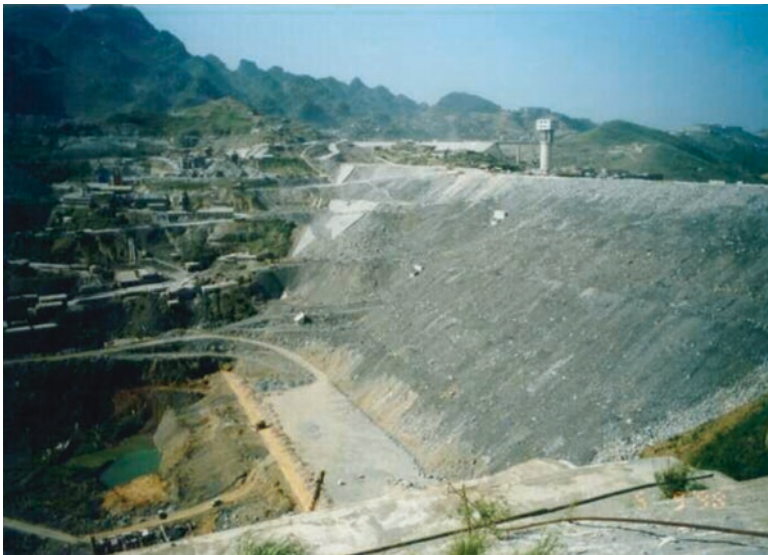
Fig. 25.6 TSQ.1 downstream view in August 1998. Detail of slope of zone III C of “mudstone”
