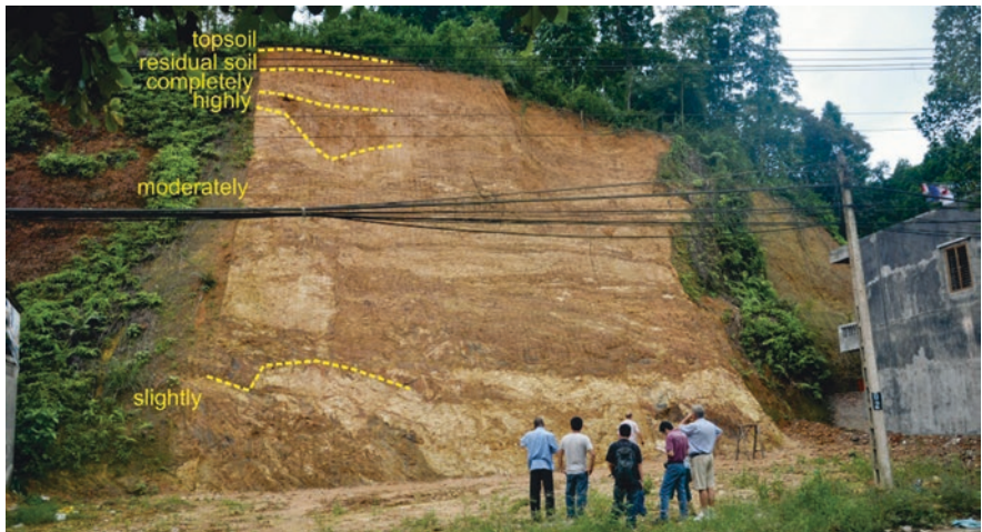
Fig. 11.6 Weathered cut slope in gneiss and schist in a tropical climate (Weathering grades follow Table 11.2 for rock masses) (Yên Bái City, Vietnam; photo courtesy D. Alkema, 2010)
