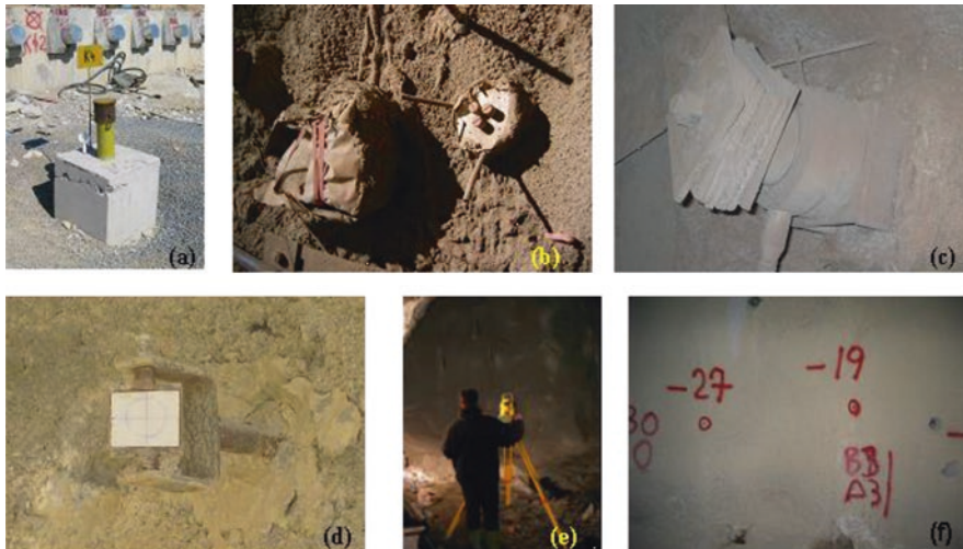
Fig. 21.13 Instrumentation and targets associated with monitoring program of Egnatia Odos; (a) monitoring well and survey target on benchmark, (b) pressure cell (left) and extensometer (right), (c) tunnel wall pressure cell, (d) tunnel wall survey target, (e) surveying the tunnel face, and (f) measurement of targets on tunnel wall (-19 denotes 19 mm of inward displacement at that target location) within Driskos Tunnel
