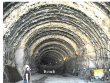
Fig. 21.15 Optical survey markers and their locations within the tunnel excavation (Grasso et al. 2003). Photo taken by author. Note that A-Phase and B-Phase are analogous to top heading and bench excavation phases respectively
