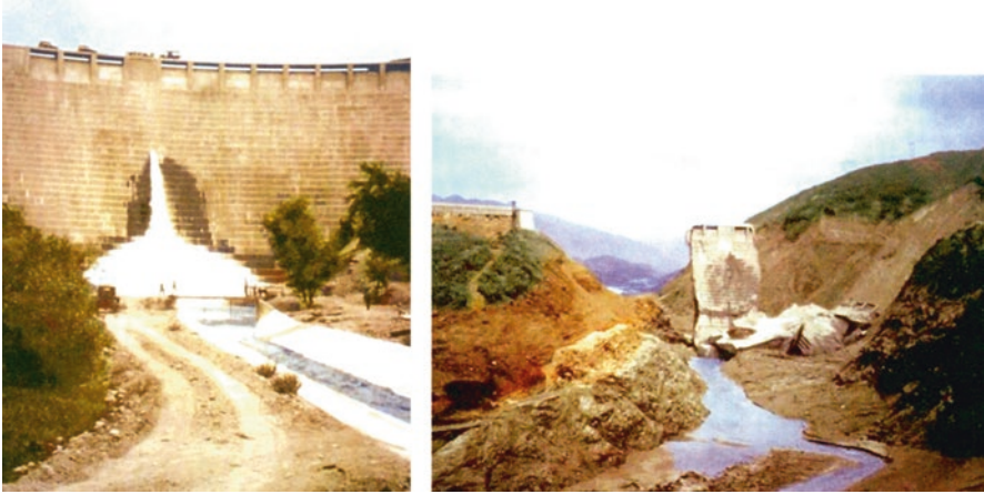
Fig. 24.9 St. Francis Dam was a curved concrete gravity arch, 209 feet high (64 m). The complete structure on the left side and the remnants on the right side (Rogers 2006)
