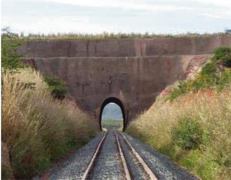
Fig. 5.12 Railroad tunnel view. (Photo E.L. Pastore)
