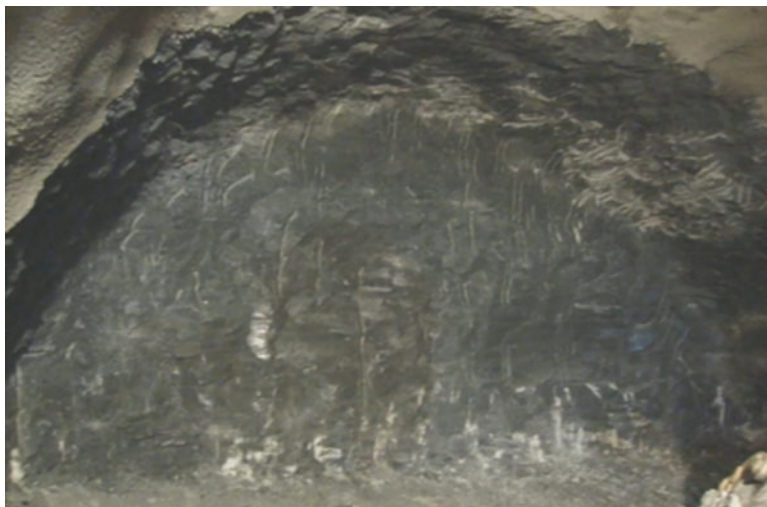
Fig. 4.32 Characteristic outcrop of mudstones at the tunnel face
