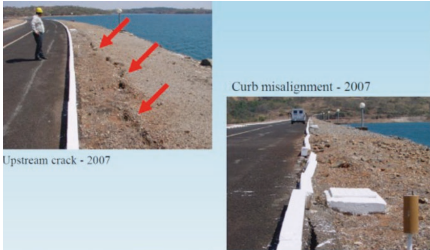
Fig. 25.3 Emborcação dam crest movements behavior after 28 years of operation
