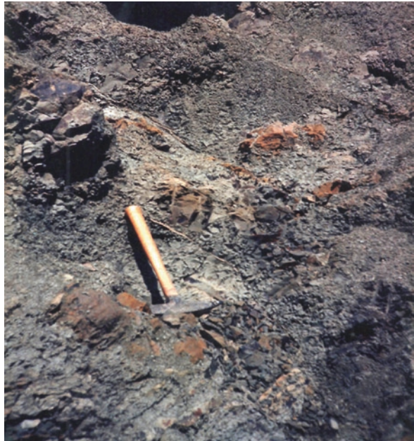
Fig. 10.4 Black shale from Ilhas Group and undifferentiated Candeias Formation, from Recôncavo sedimentary basin, Bahia state, Northeast Brazil. It can be seen the effects of disaggregation (slaking) of rock, due to its explosion to weathering in a cut-slope
