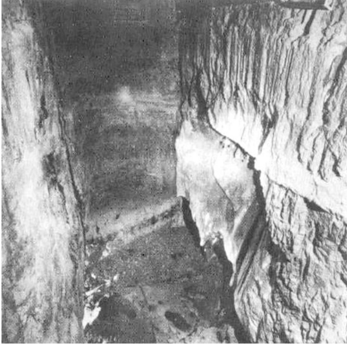
Fig. 20.20 Accident occurred in a surge chamber of Cahora Bassa (Rocha 1975)
