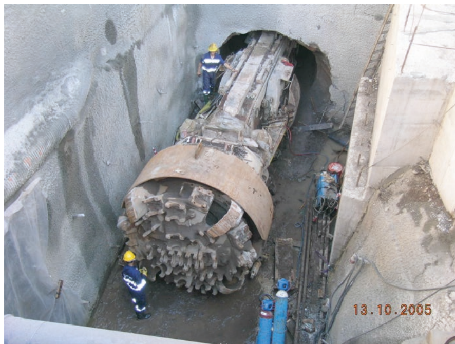
Fig. 20.4 TBM used at Covão tunnel
