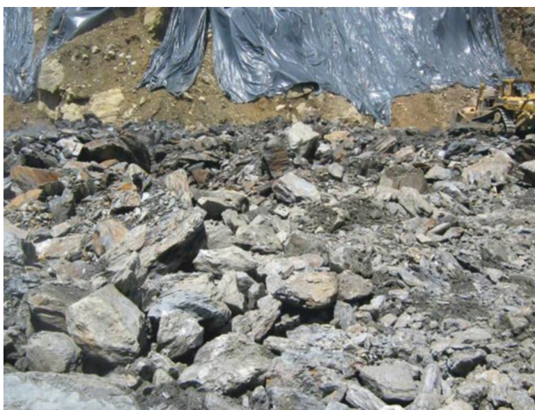
Fig. 25.17 Zones 3D & 3C. Dam fill at el. 555.7 70% IIB + 30% IIA
