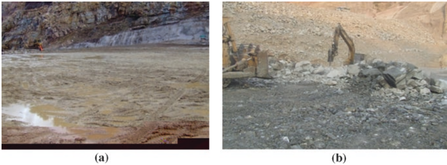
Fig. 25.24 Soft sandstones materials at dam center zone (Moll and Straubhaarr 2011)
