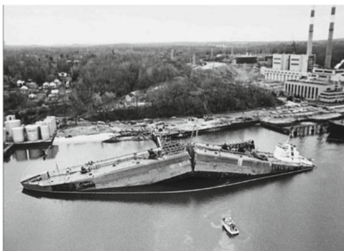
Fig. 6.26 Liberty ship that failed while docked in calm waters during a cold winter day
