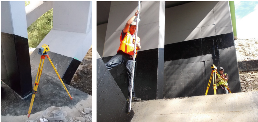
Fig. 3. Digital level station with the automatic recording of results and surveying of vertical displacements of the arch girders at their springing points and interfaces with the foundations.
