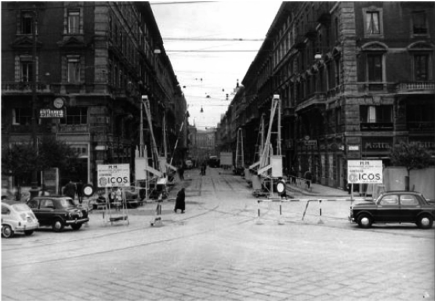
Fig. 1. Diaphragm wall works in Milan from 1956 (Quelle: Wikipedia)
