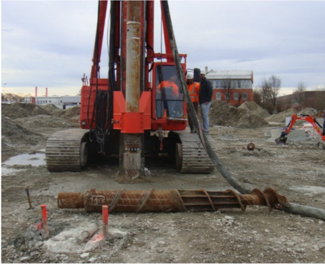
Fig. 7. Displacement auger used to install the CMC piles.
