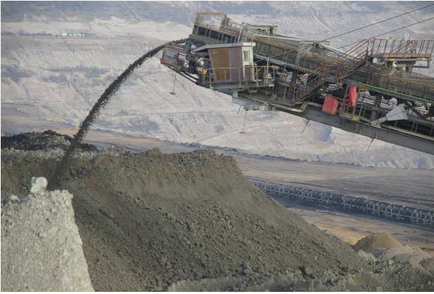
Fig. 2. Deposition of the excavated soil.
