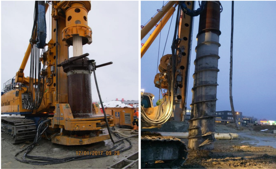
Fig. 6. BAUER BG46 with: casing oscillator and water inflow (left) and ring auger to eliminate the skin friction in the cover layer (right).
