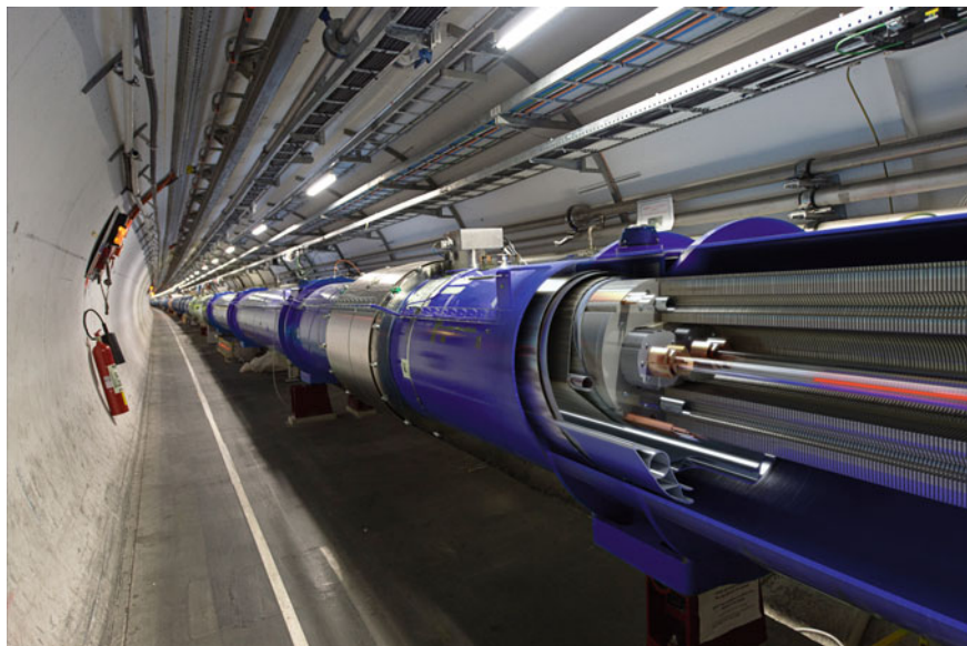
Fig. 1 LHC Tunnel. Courtesy of CERN
