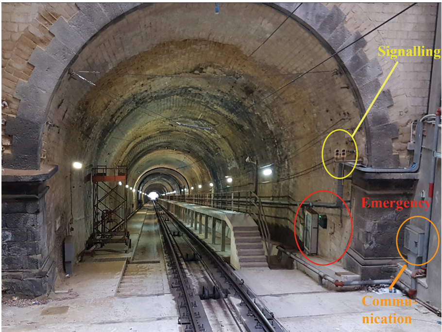
Fig. 1. Signalling, communication and emergency components funicolare between Petraio and Fuga [own elaboration]
