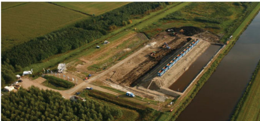
Fig. 19 Levee section under test, Netherland. Courtesy of Deltares
