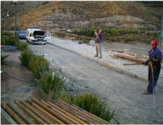
Fig. 28 Installation of long-gauge strain sensors in a borehole
