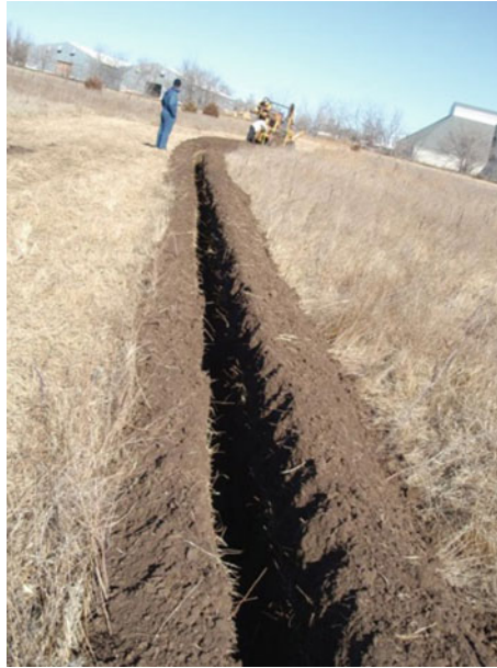
Fig. 24 Distributed strain sensor installation in a trench
