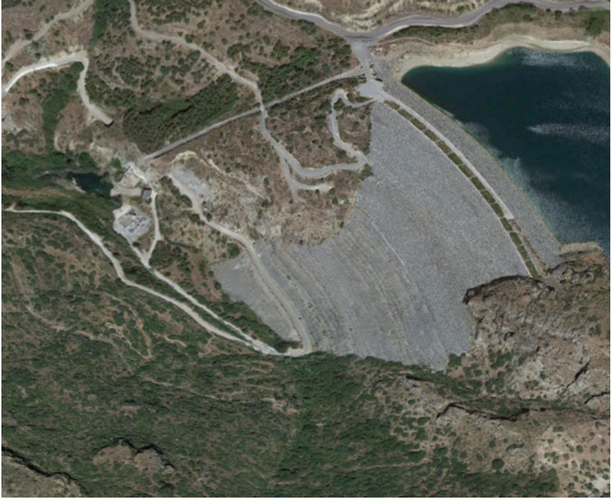
Fig. 27 Canales Dam, Spain
