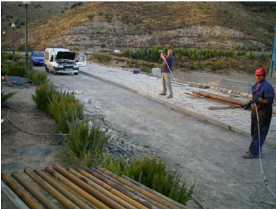
Fig. 28 Installation of long-gauge strain sensors in a borehole
