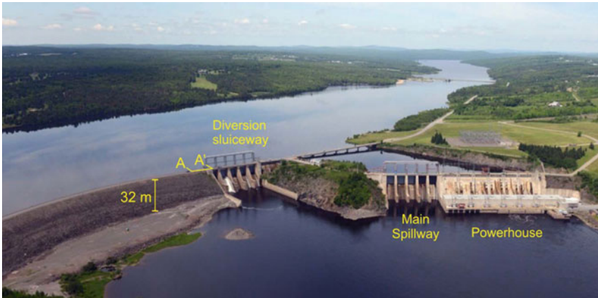
Fig. 2 Aerial photo of the Mactaquac hydroelectric generating station, with its 500 m long zoned rockfill embankment dam
