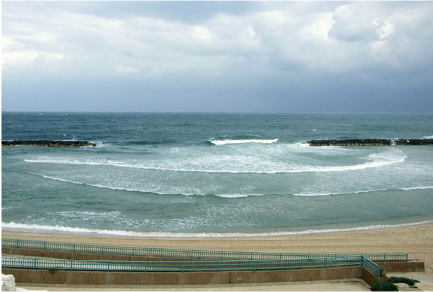
Fig. 5.16 Ocean waves diffract as they pass through an opening in a breakwater (Dmitris1 ( https://commons.wikimedia.org/wiki/File:BreakWaterDiffraction_Ashkelon1.jpg ), https://creativecommons.org/licenses/by-sa/4.0/legalcode )
