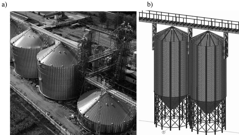
Fig. 1. Steel containers for storage of grain: a general view of the vertical silos Lubnymash (a) https://lubnymash.com ; calculation scheme of capacitance; calculations of MSC (b)
