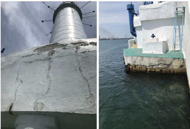
Fig. 2. Nowadays condition of the Vorontsov Lighthouse
