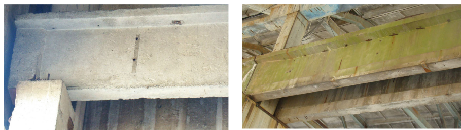
Fig. 1. Crane beams BKNB6-2c (on the left) and BKNB12-1c (on the right)
