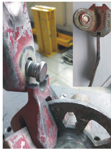
Fig. 4. Failure of the joint elements.
