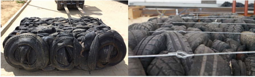
Fig. 1. Tyre bale (left) and galvanized steel wires spanning tyre bales (right)
