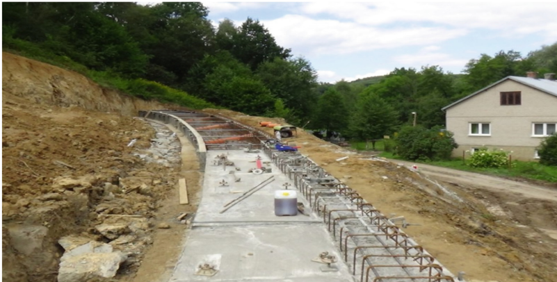
Fig. 5. Realization of the landslide stability solution with piles and anchors.
