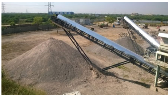
Fig. 1 C&D waste processing unit in Ahmedabad (Source Development Alternatives)
