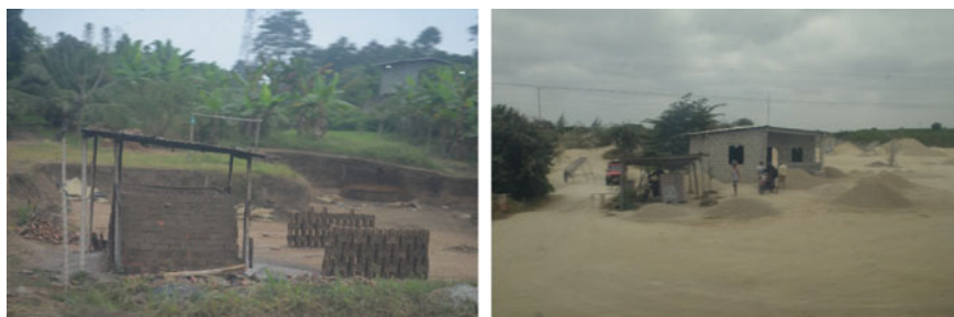
Fig. 6 Artisanal brick production from local clay in Guayas Province (left) and artisanal sand extraction (right) in Santa Elena Province in Ecuador
