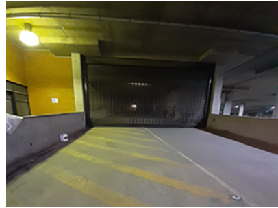
Fig. 4. Exit point of the facility.
