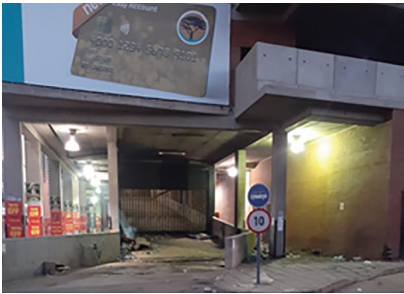
Fig. 3. Entry point into the facility.
