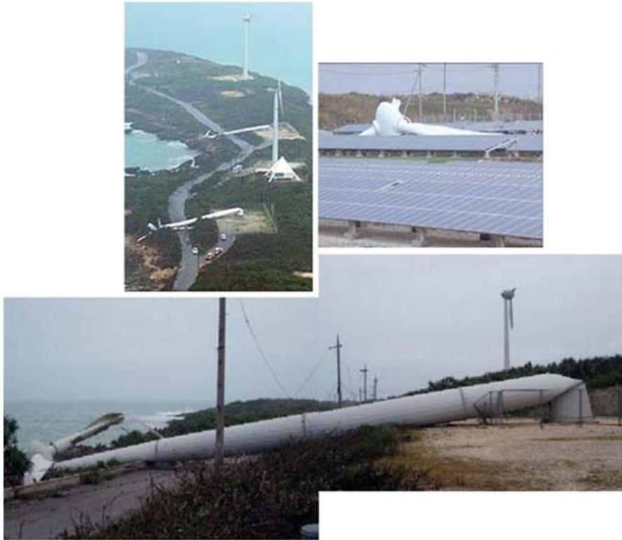
Fig. 4.5 Wind turbine destroyed by strong typhoon in Miyako Island
