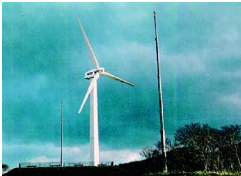
Fig. 4.2 NEDO 500 kW wind turbine at Cape of Tappi in Aomori
