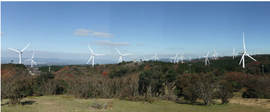
Fig. 4.9 Shin-Aoyama-Kogen Wind Farm, in Mie pref., 80 MW (the largest in Japan), Hitachi 2 MW × 40 units, start operation in February 2017. (Courtesy of Aoyama Kogen wind farm)
