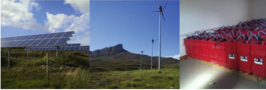
Fig. 7.19 The main components of the Isle of Eigg (Scotland) wind-based hybrid Power station
