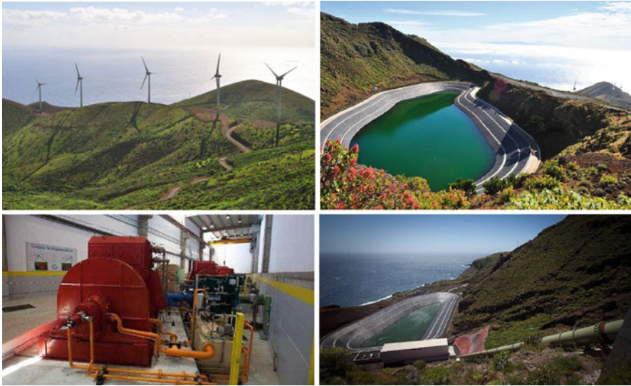
Fig. 7.17 The main components of the El-Hierro wind-based hybrid power station
