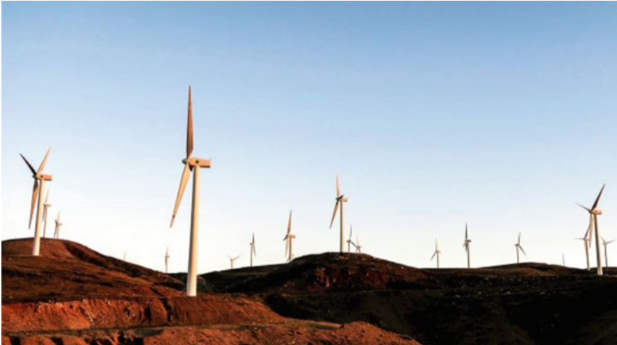
Fig. 5.9 View of Fujeij wind farm
