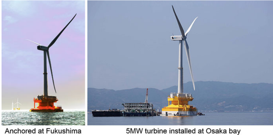
Fig. 4.10 Hitachi 5 MW floating offshore wind turbine. (Courtesy of Fukushima FORWARD)
