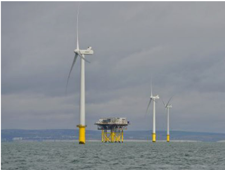
Fig. 2.9 Rampion wind farm, 13–20 km off the south coast of England, was completed in 2018. It comprises 116 wind turbines, each with a rated output of 3.45 MW, a rotor diameter of 110 m, and a hub height of 80 m. The projected output is 1.4 TWh/year. The photograph shows the substation where the power is marshalled. (Photo courtesy of Rampion Offshore Wind)
