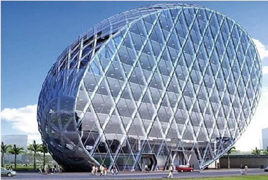
Fig. 1 A typical diagrid structure [4]
