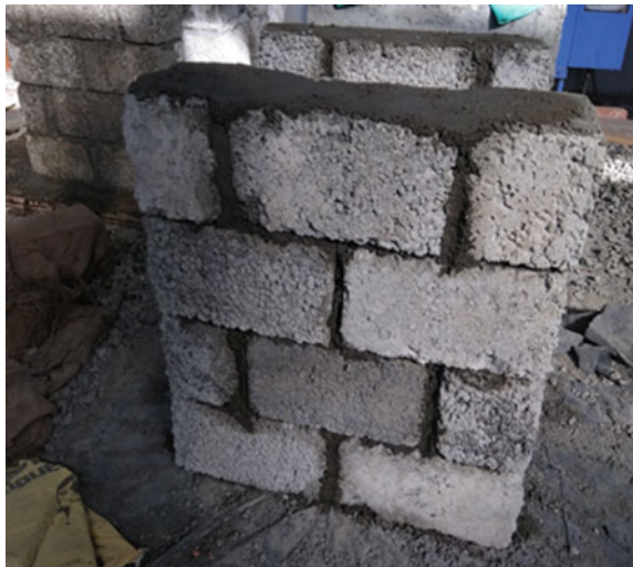
Fig. 2 concrete block panels
