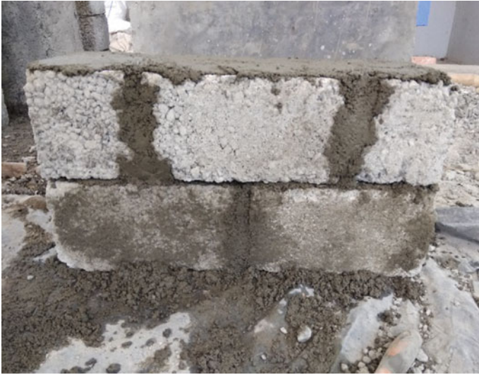
Fig. 1 Casting of concrete block panels
