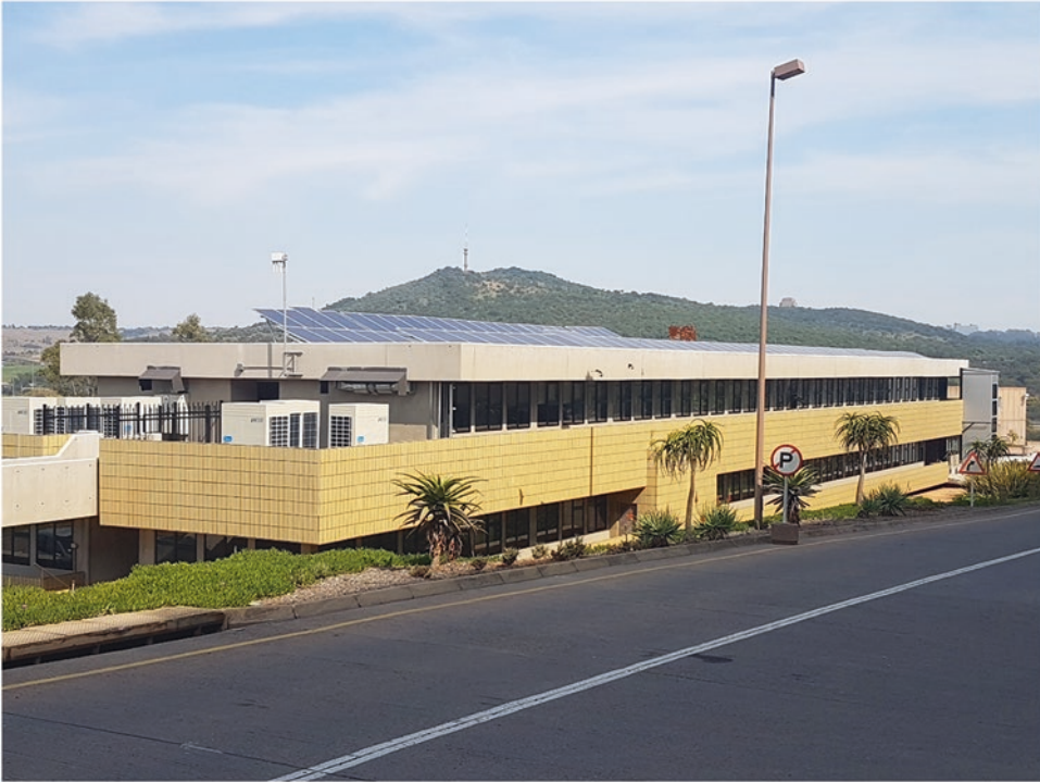
Fig. 3.7 RR Maluleka Building Rooftop Solar Farm (Muckleneuk) (Source: Author)
