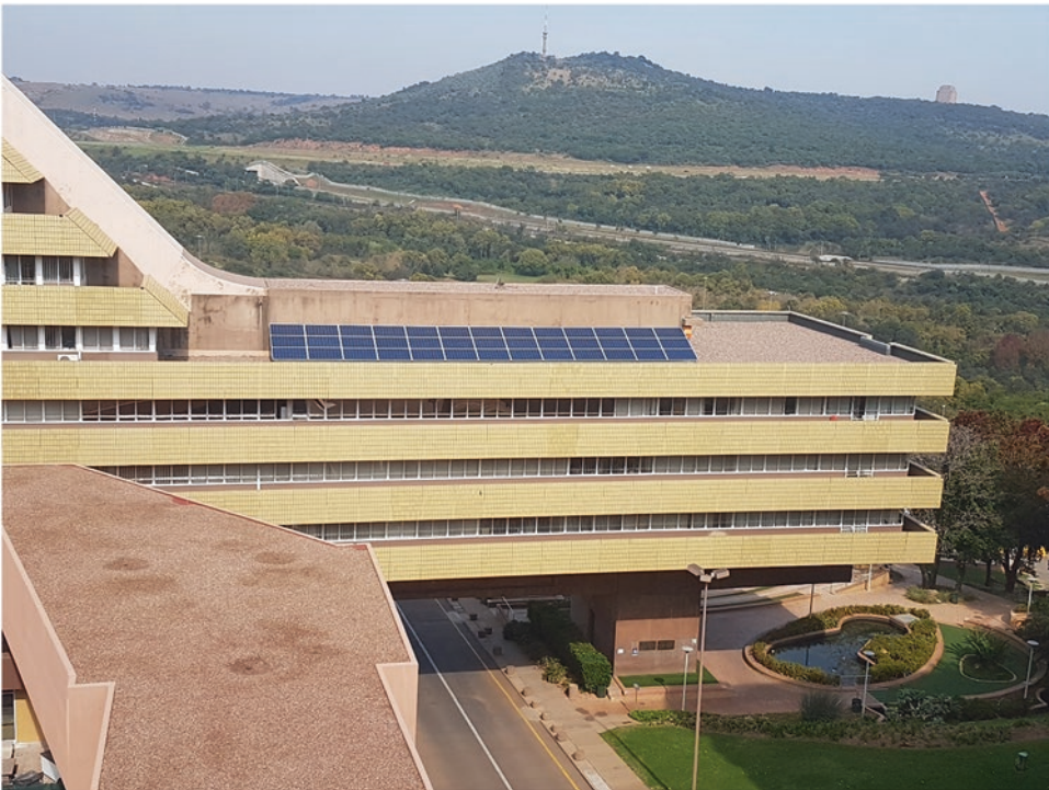
Fig. 3.8 OR Tambo Building Rooftop Solar for the eGarden (Muckleneuk) (Source: Author)
