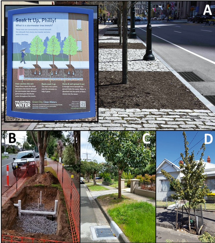
Fig. 17.3 Trees in stormwater control measures: a linear planting of trees in an SCM trench along a street in downtown Philadelphia, USA (a); a small SCM trench of gravel during construction (b) and after construction (c) in Melbourne, Australia; and a simple kerb-cut SCM where a tree is planted into the small biofilter sand rain garden in Melbourne, Australia (d). (Photo credits: DE Carlyle-Moses (a), C Szota (b and c), and J Thom (d))
