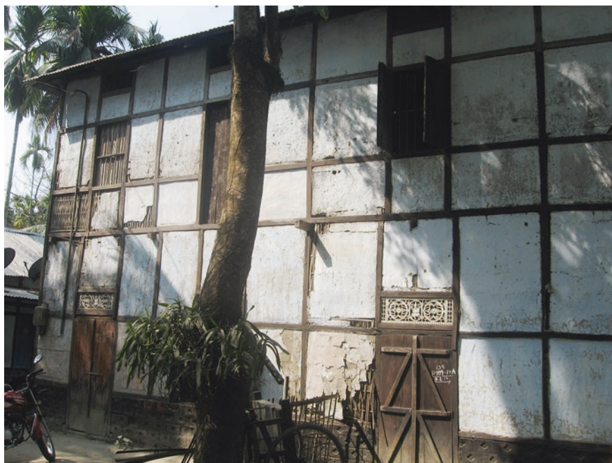
Fig. 9.11 Ikra wall panels with mud plaster
