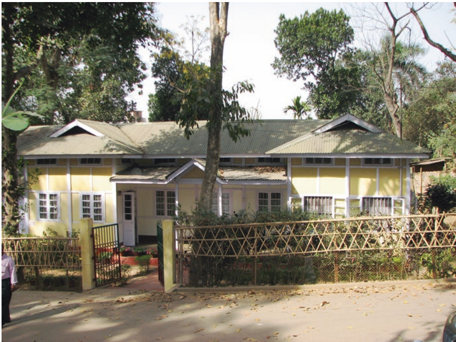
Fig. 9.7 Single-storeyed Ikra structure. (Photo: Author)
