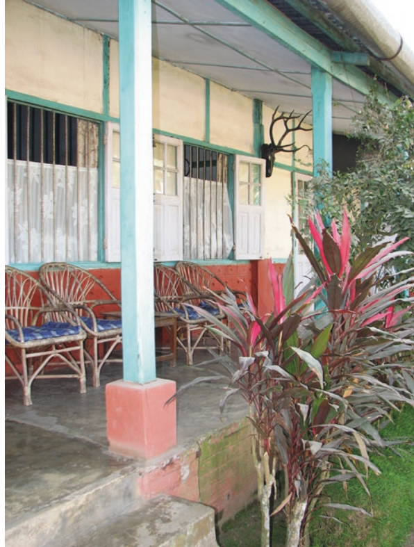
Fig. 9.12 Brick masonry pedestals supporting the vertical timber posts
