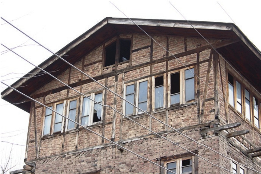
Fig. 9.5 Vertical and horizontal wooden frame members on the upper floor with diagonal framing at the corners of both faces of the building. (Photo: Author)
