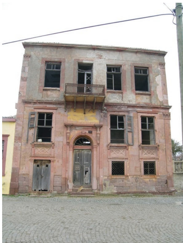
Fig. 15.37 Asymmetric facade, Ayvalık Street
