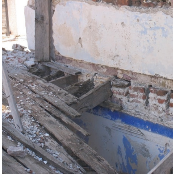
Fig. 15.66 The wooden flooring with wooden beams
