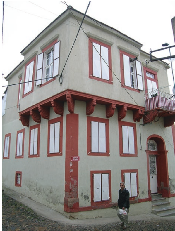
Fig. 15.36 Corner house, Şeref Street
