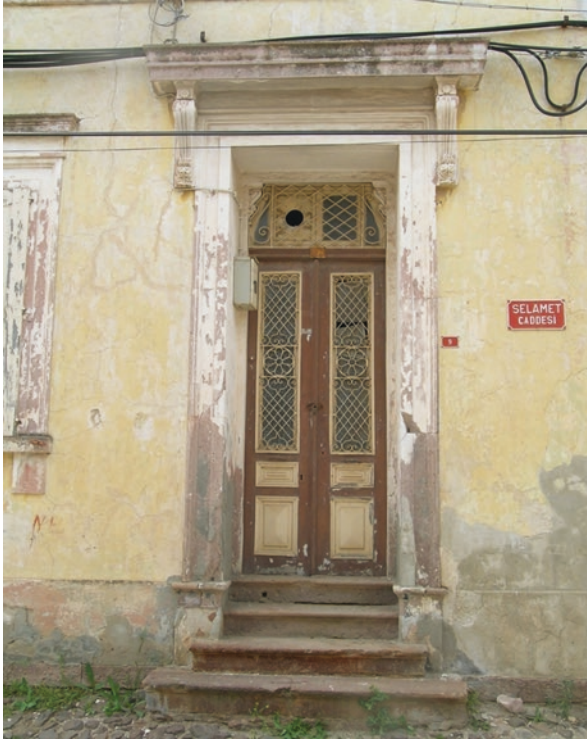
Figs. 15.46 and 15.47 Main doors protected within a niche
