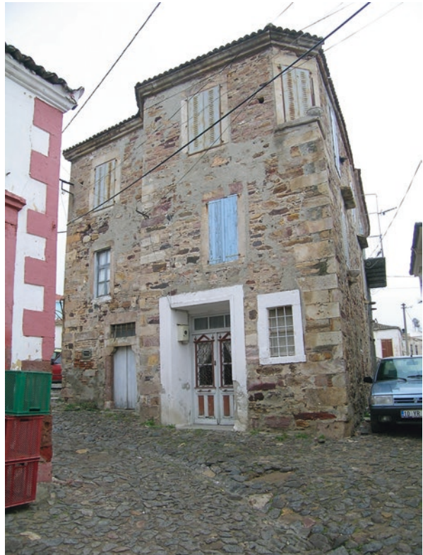
Fig. 15.61 The walls are built with local stone
