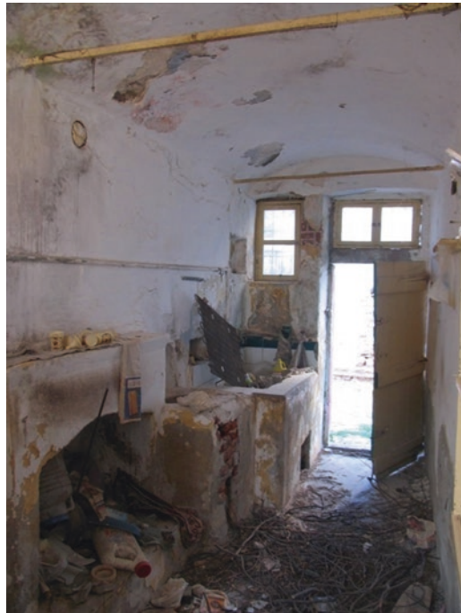
Figs. 15.67 and 15.68 The ceilings of the ground floors
