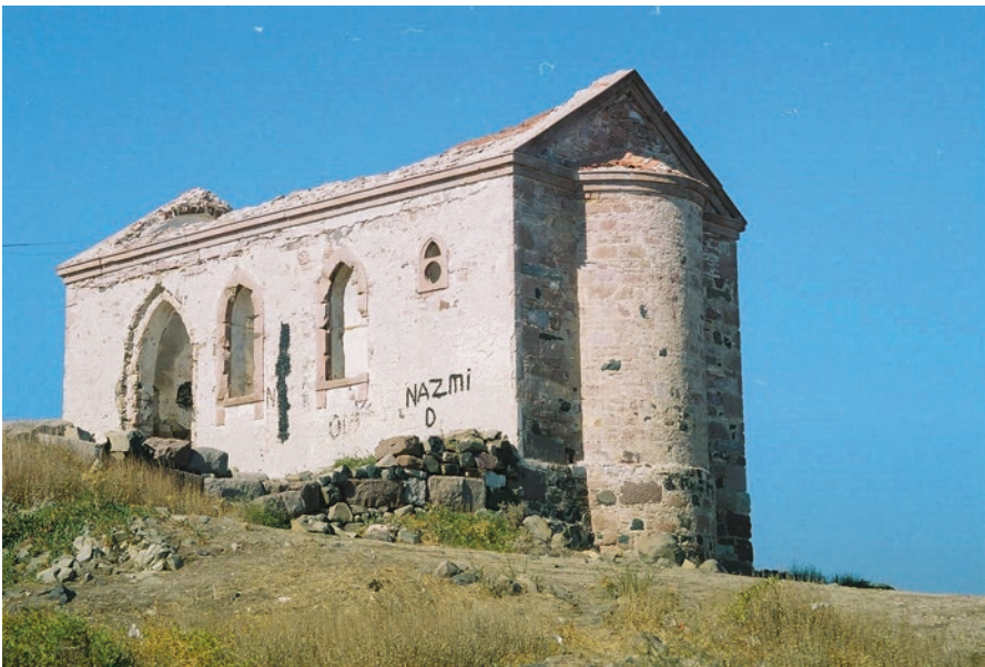
Fig. 15.13 St Iannis Church, before the restoration, Aşıklar Hill
