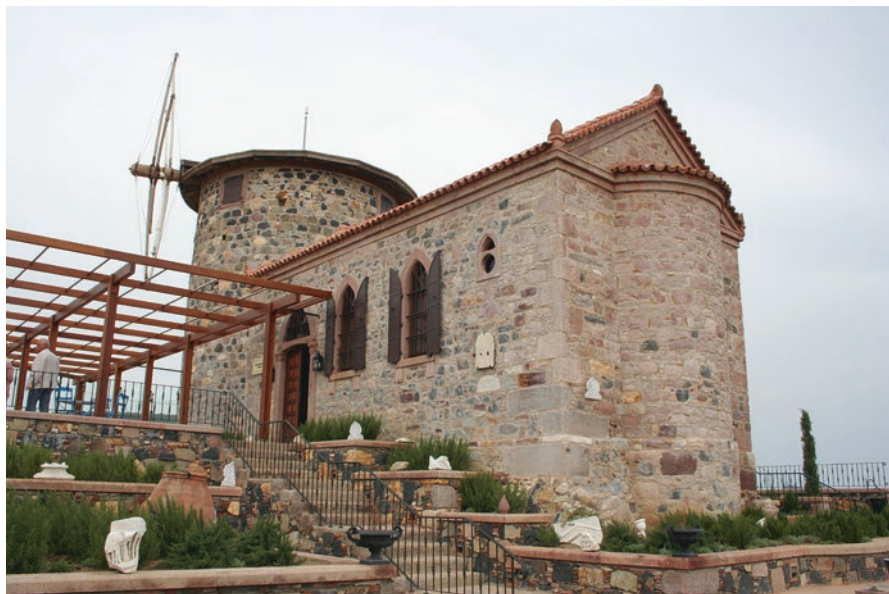
Fig. 15.14 St Iannis Church, after the restoration
