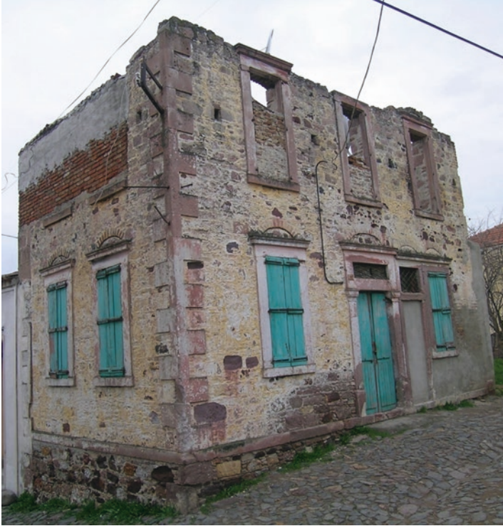
Fig. 15.55 Exterior walls are made up of rough stone
