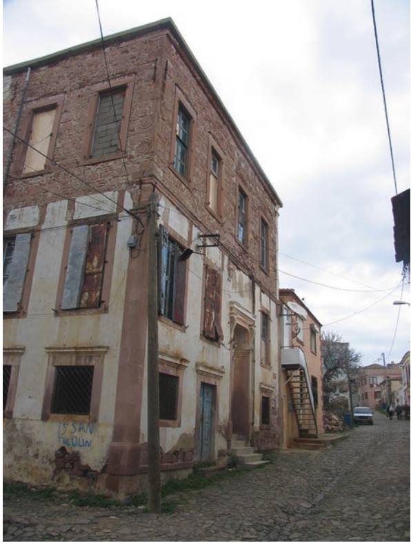
Fig. 15.56 Sometimes exterior walls of the upper floors are made up of brick
