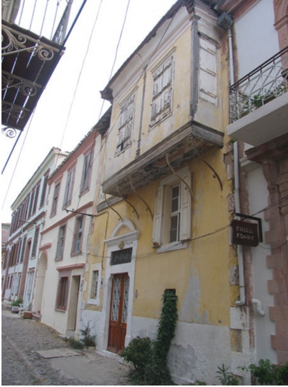
Figs. 15.51, 15.52, 15.53, and 15.54 Different projections on street and side facades with iron supports and stone consoles
