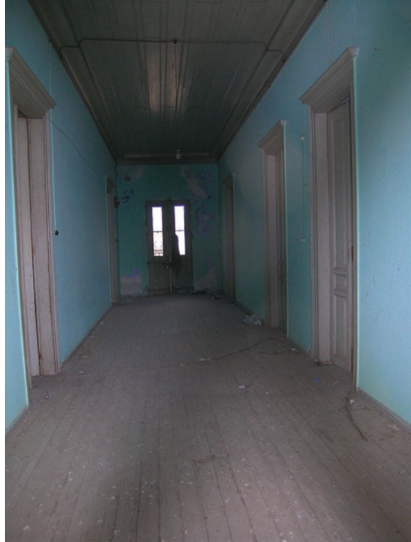
Fig. 15.29 The narrow hall provides access to the rooms
