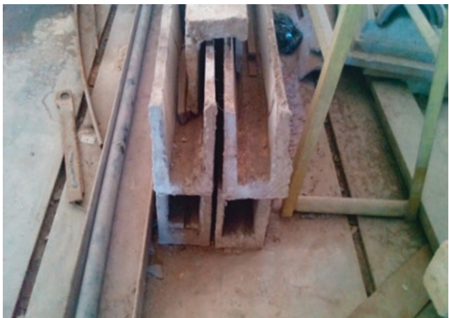
Fig. 14.9 Appropriate disappearing beam formwork. (Source: Moses 2015)
