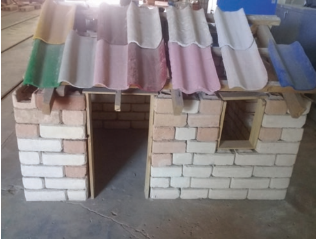
Fig. 14.11 Construction model showing: soil-cement interlocking brick wall, appropriate disappearing beam formwork and sisal concrete roofing tiles on timber truss members. (Source: 2018 Survey at NHBRA)
