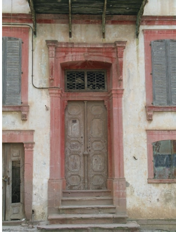
Fig. 15.40 The main entry door
