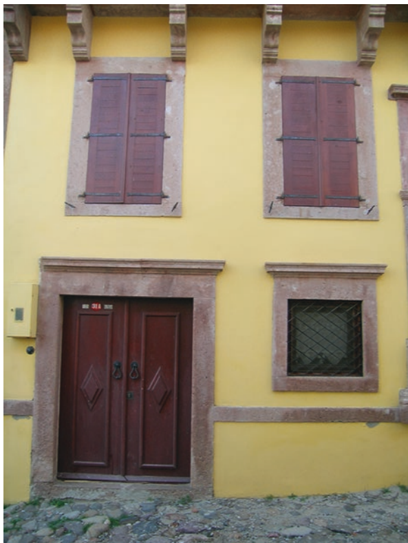
Fig. 15.45 Square windows of ground floor, rectangular windows of upper floors
