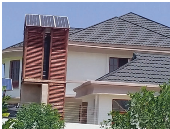
Fig. 14.15 Use of solar energy in buildings in Mbweni – Dar es Salaam. (Source: 2018 Survey)
