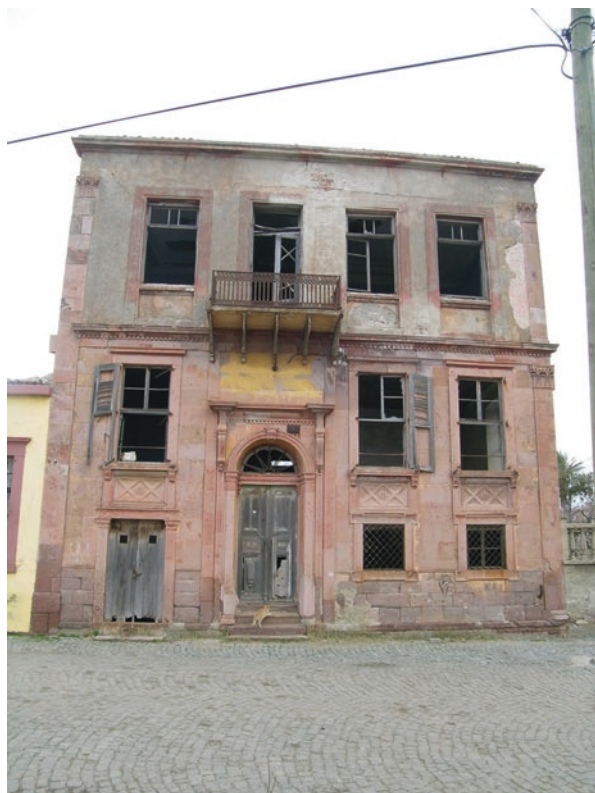
Fig. 15.37 Asymmetric facade, Ayvalık Street
