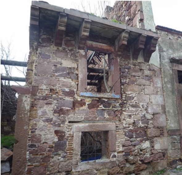
Figs. 15.59 and 15.60 The rough “Sarimsak” stone walls
