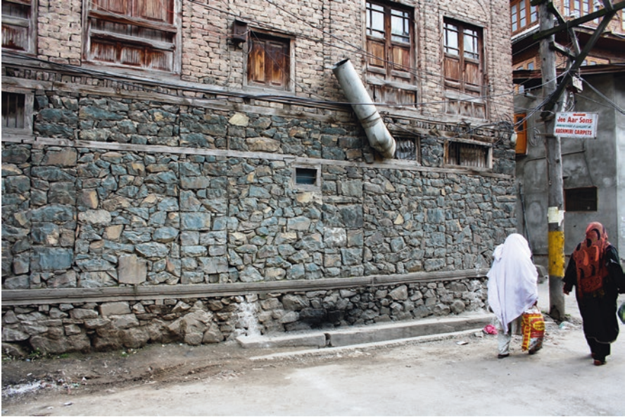
Fig. 9.2 Use of large stones and continuous wooden plinth bands. (Photos: Author)
