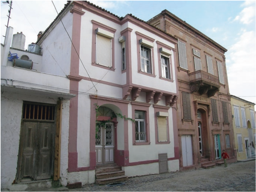
Fig. 15.34 Street facades of the houses, Selamet Street
