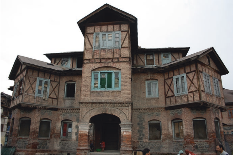
Fig. 9.4 Two-storeyed house, rectangular in plan in the ground floor with diagonally placed room projections on the upper floor. (Photo: C.V.R Murty)
