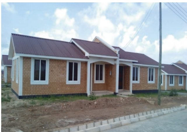
Fig. 14.4 Kigamboni residential house built with soil-cement interlocking bricks. (Source: Moses 2015)
