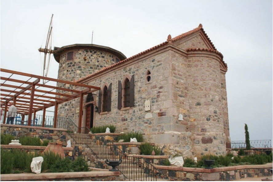
Fig. 15.14 St Iannis Church, after the restoration
