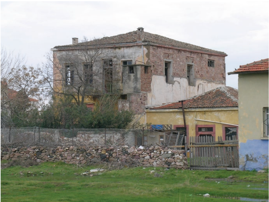
Fig. 15.35 Back facade of the Cunda house
