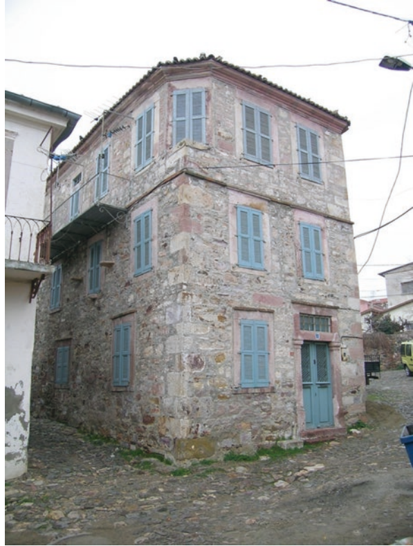
Fig. 15.42 Unplastered facade
