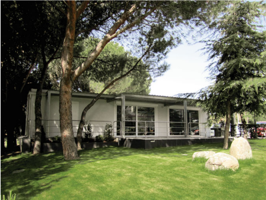
Fig. 13.1 Smart House Living Lab facilities
