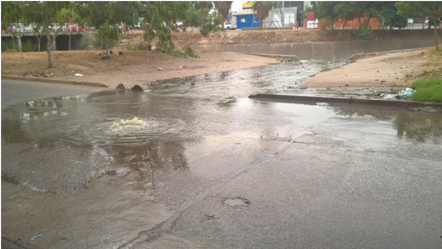
Fig. 21.3 Urban sewer is throwing wastewater and discharging into an urban drain ( picture Otoniel Carranza)
