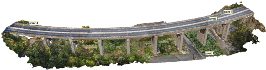
Fig. 13. Annunziata Viaduct 3d model
