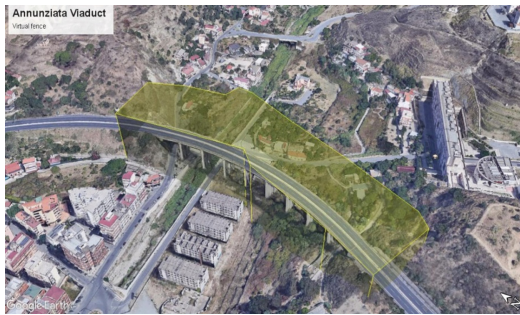
Fig. 8. Geo-fence around Annunziata Viaduct for delimitation of aerial space for survey
