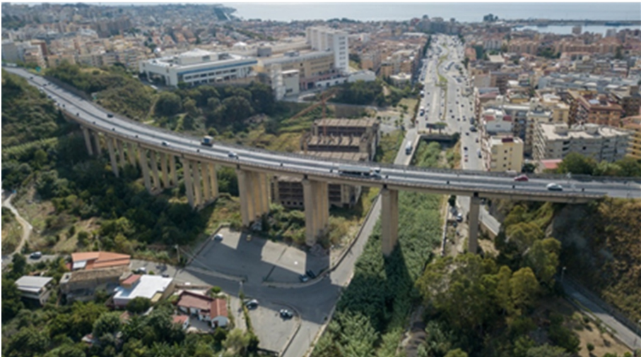
Fig. 3. Aerial view of highway viaduct Annunziata, Reggio Calabria, Italy
