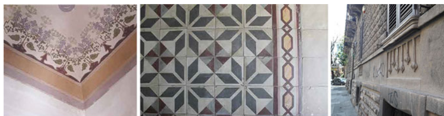
Fig. 6 Details of the frescoed vault, the flooring in cement tiles and the basement of the front in via XX Settembre
