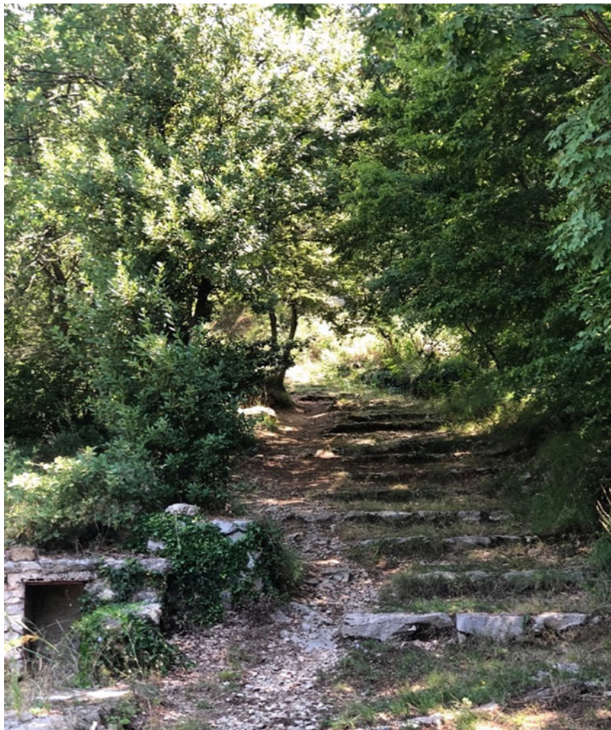
Fig. 6 Park avenue Source authors' picture
