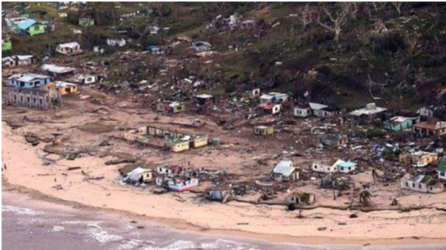
Fig. 4 Picture of Vatulale Village, north-eastern extremity of Koro Islands after TC Winston. Koro was one of the most affected small islands in Fiji, where most of the damages were caused by strong wind (185 km/h) and the storm surge. Source Fiji National Disaster Risk Management Office (n.d.)
