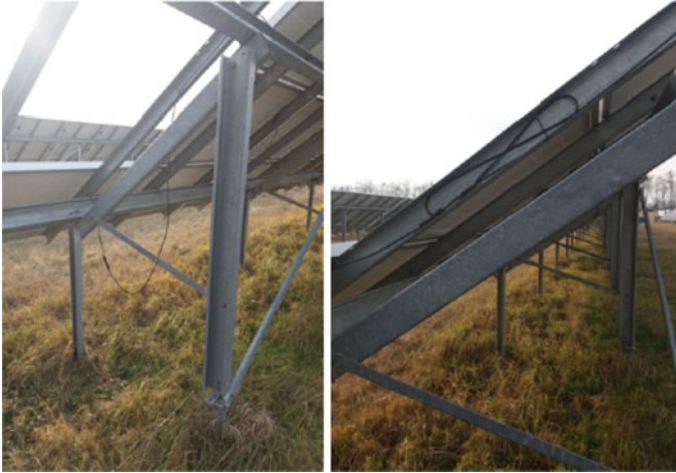
Fig. 11.2 Cables arranged on the structure
