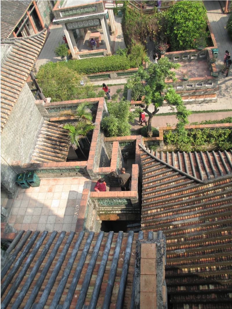
Fig. 2. The stairwell vent, the courtyard vent and the patio vent of the Ke Building in Ke Garden.
