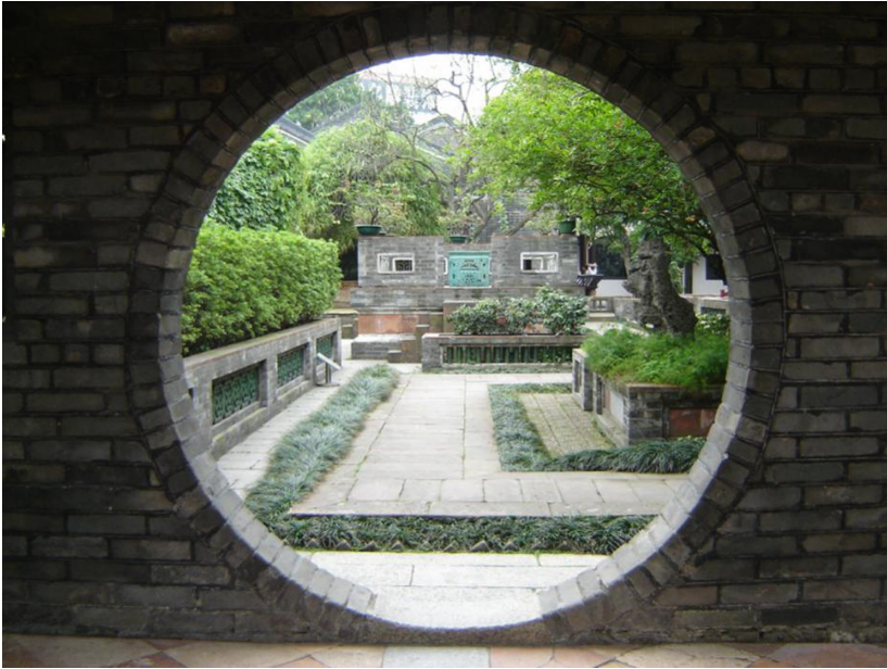
Fig. 8. The permeable materials of Ke Garden in Dongguan: big step bricks indoors and mosaic bricks, red sandstones and grass belts outdoors. (Color figure online)
