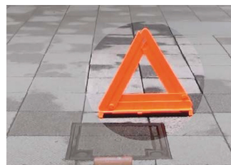
Fig. 2. Incorrect installation of stop indicator
