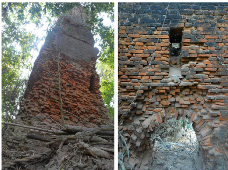
Fig. 6 Sāmālia GTS tower station showing external façade (left) and internal view of brickwork, doorway and window opening with scale rule (10 mm gradations) (right)
