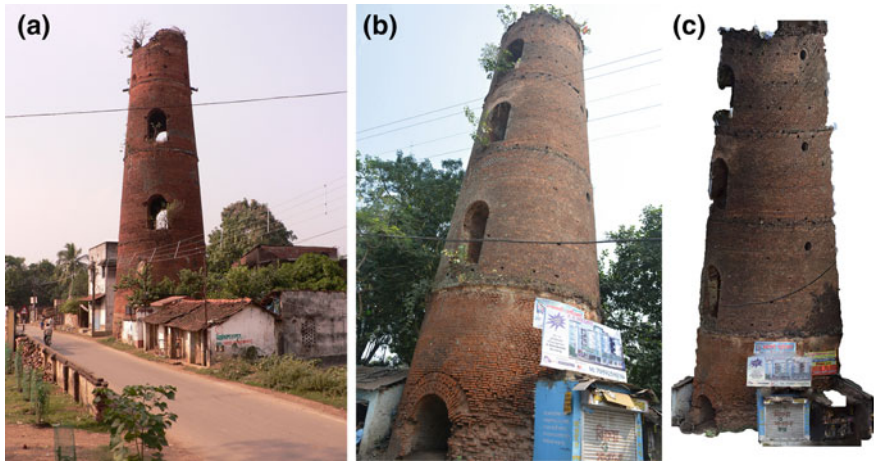
Fig. 5 Cylindrical GTS tower stations reusing earlier semaphore towers at Dilākās (a), and at Nibria (b) including a Structure from Motion (SfM) visualization of Nibria (c)
