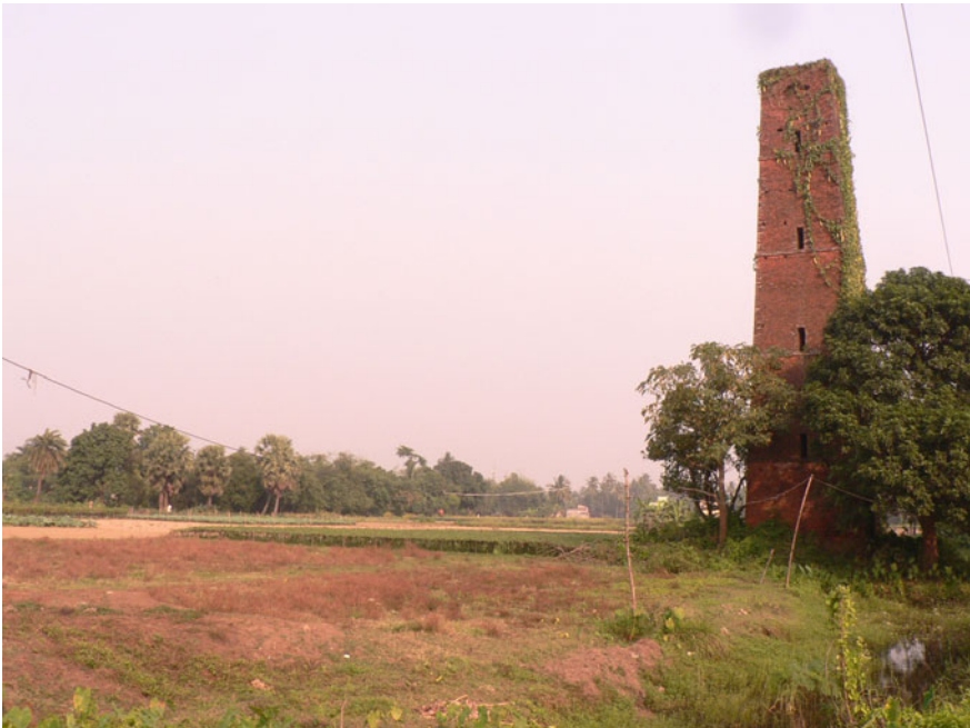
Fig. 4 The GTS tower station at Bhola on Singur to Tarakeswar road
