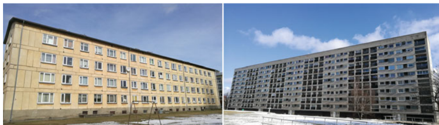
Fig. 16.3 Large block (left) and brick (right) apartment buildings in Tallinn housing estates
