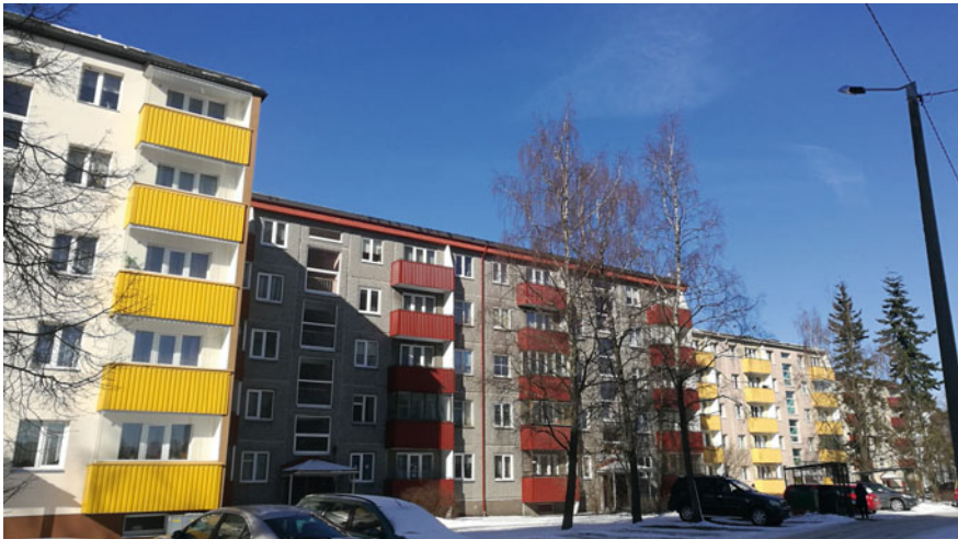
Fig. 16.11 Various façade treatments on adjacent apartment buildings
