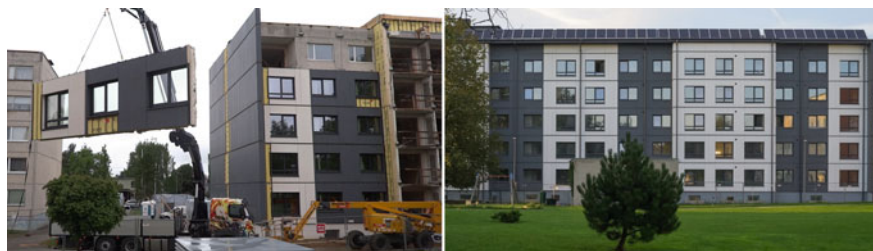
Fig. 16.12 Installation of modular wall panels (left) and the finished building (right)
