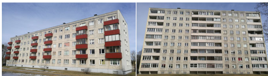
Fig. 16.4 Large-panel apartment buildings in Mustamäe: 1–464A (left) and 1–464D (right)
