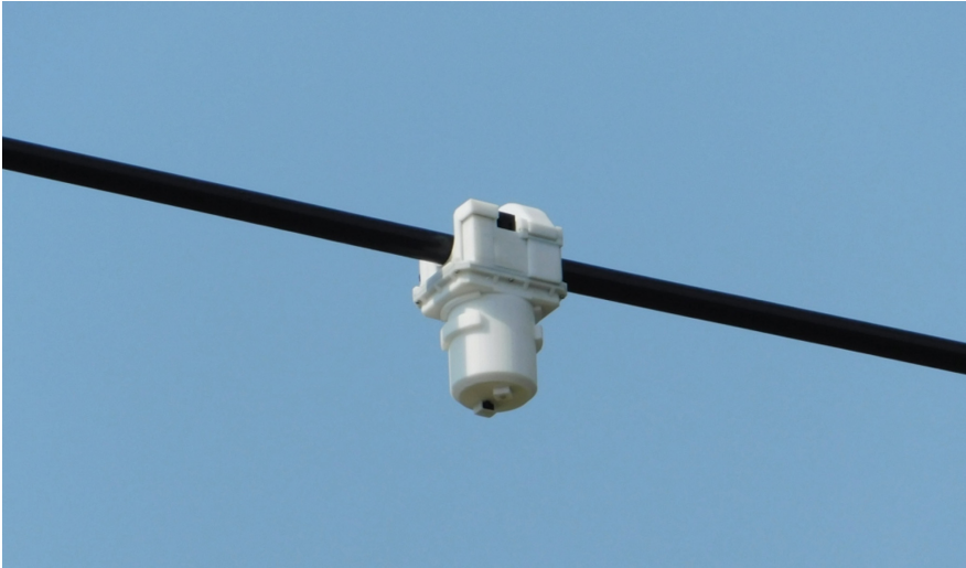
Fig. 9. The client node on high-voltage cable after installation
