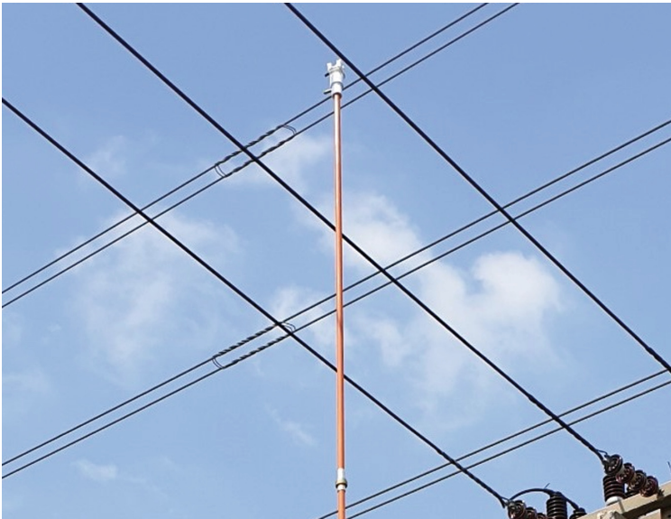
Fig. 8. The disconnect stick for installation
