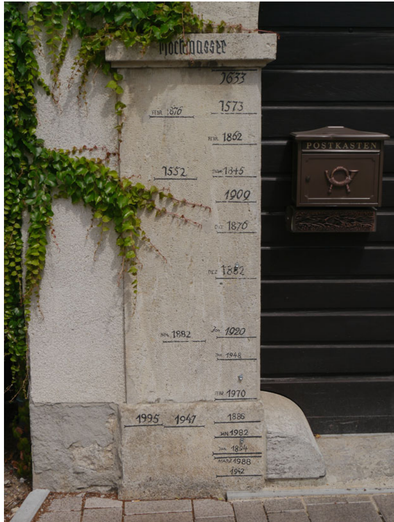
Fig. 10.15 Compilation of 20 historic flood levels of the River Main at Randersacker/Germany dating back up to AD 1552. Photograph Herget
