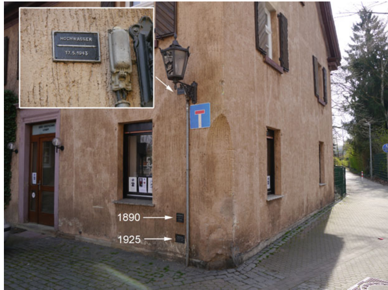
Fig. 3.6 Dam-break flood level on 17th of May 1943 in comparison with previous natural flood levels as shown by flood markers on a building in Schwerte
