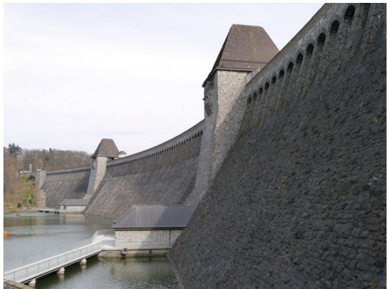
Fig. 3.2 Air side of the recent dam wall of the Möhne Reservoir; the visible water surface is a compensation basin on the downstream side of the dam wall
