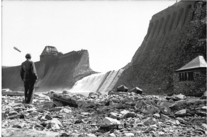
Fig. 3.4 Destroyed dam wall of the Möhne Reservoir, 17 May 1943 (Bundesarchiv 101I-637-4192-23/Schalber—reprinted by permission of the publisher)
