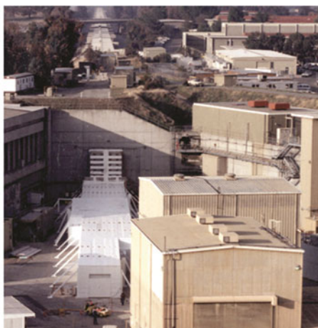
Fig. 2 The X-ray beam path for LCLS, as envisioned in 1993 (Tatchyn and Pianetta 1993). The top schematic shows the path of the X-ray beam as it is deflected out of the final focus test beam (FFTB) enclosure. The photograph on the bottom shows the FFTB enclosure ( white concrete block structure with diagonal braces) and utility buildings which might have housed experiment stations to the bottom . At the top of the photograph, the SLAC linac klystron gallery is visible, receding into the distance
