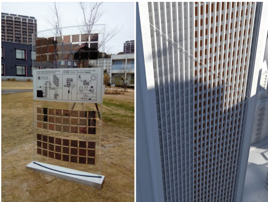
Fig. 10.17 (left) Curved glass façade element in Nagasaki, Japan with 72 printed perovskite modules (right) Visualization of a BIPV application: perovskite modules integrated into windows of a skyscraper. Courtesy of Saule Technologies
