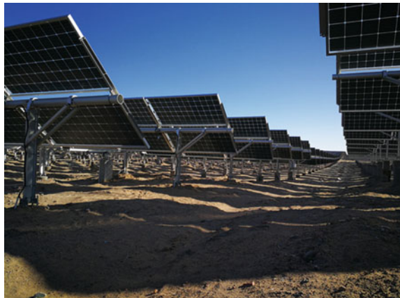
Fig. 5.9 Photograph of a large scale 20 MWp PV power plant installed by LONGi in Golmud, China, applying bifacial PERC+ solar cells in combination with one-axis trackers thereby maximizing the energy yield from the modules front and rear side [91]
