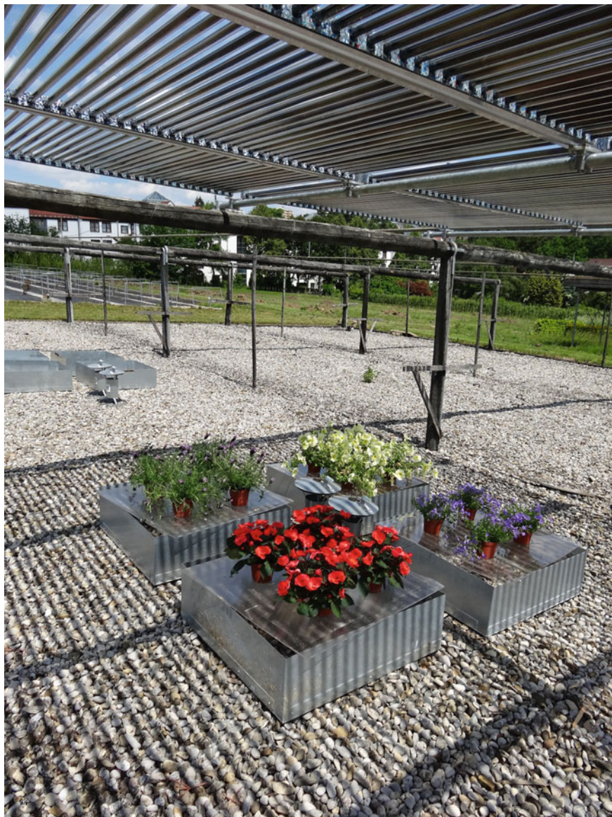
Fig. 11.13 ATPV power Pergola build in 2014 in Weihenstephan, Freising
